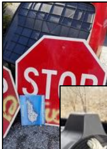
Removing Signs and Clearing Roadside Trash
