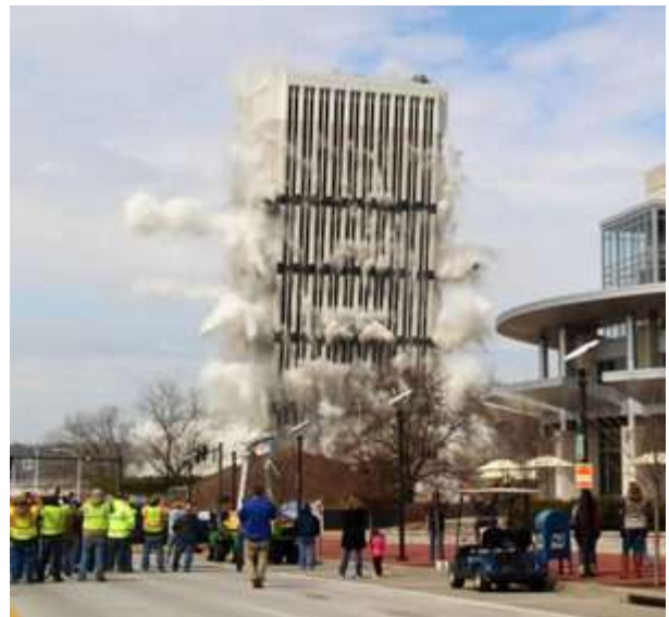
Tower Demolition in March 2018
