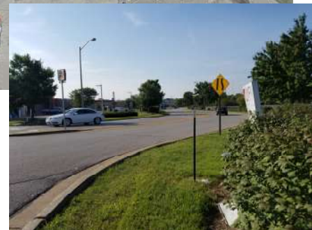
Initial improvement concept (above); view along Leonardwood Drive SB at inbound merge area with landscaping limiting sight distance for turns from cross-streets (right).
